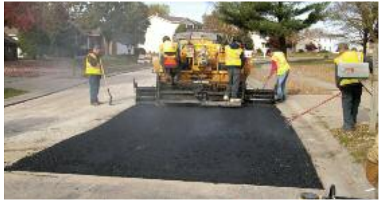
A crew works on a road patch in Crowne Pointe.
